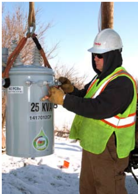
First installation of a FR3 fluid-filled transformer at ComEd in March 2008.
