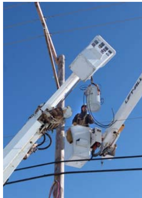
First installation of a FR3 fluid-filled transformer at ComEd in March 2008.
