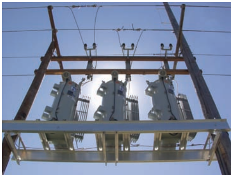
Single-phase step voltage regulator configuration.
