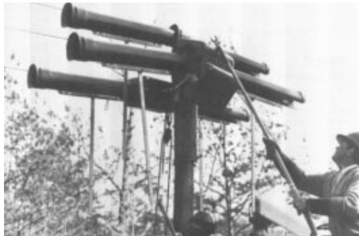
Figure 23. Coupler type line guards assure safety against contact with energized wires as crew installs stand-off insulator covers to complete protection on armless construction.
