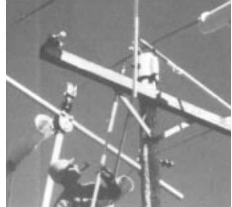
Figure 31. Pole top cover adds safety when insulator ties are removed or new wire is being installed. Line guards were installed on each side of work area.
