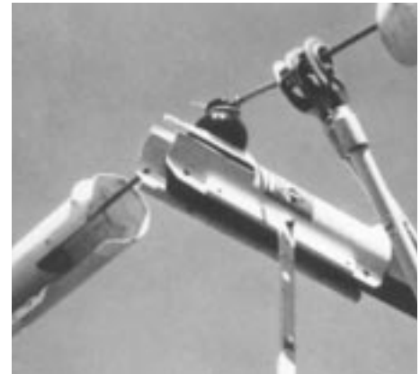
Figure 32. Crossarm guard prevents arm contact when insulator tie is removed from outside conductor. Line guards protect operator from contact with wire.
