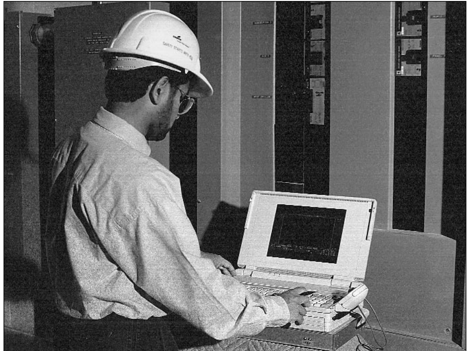
Figure 1. Experienced engineers using sophisticated measurement equipment conduct on-site harmonic measurements.
