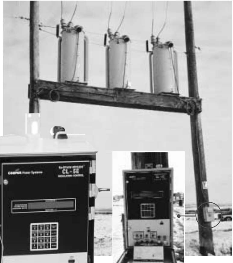
Cooper CRA controlling pole-mounted Siemens regular outside Boise, Idaho.
